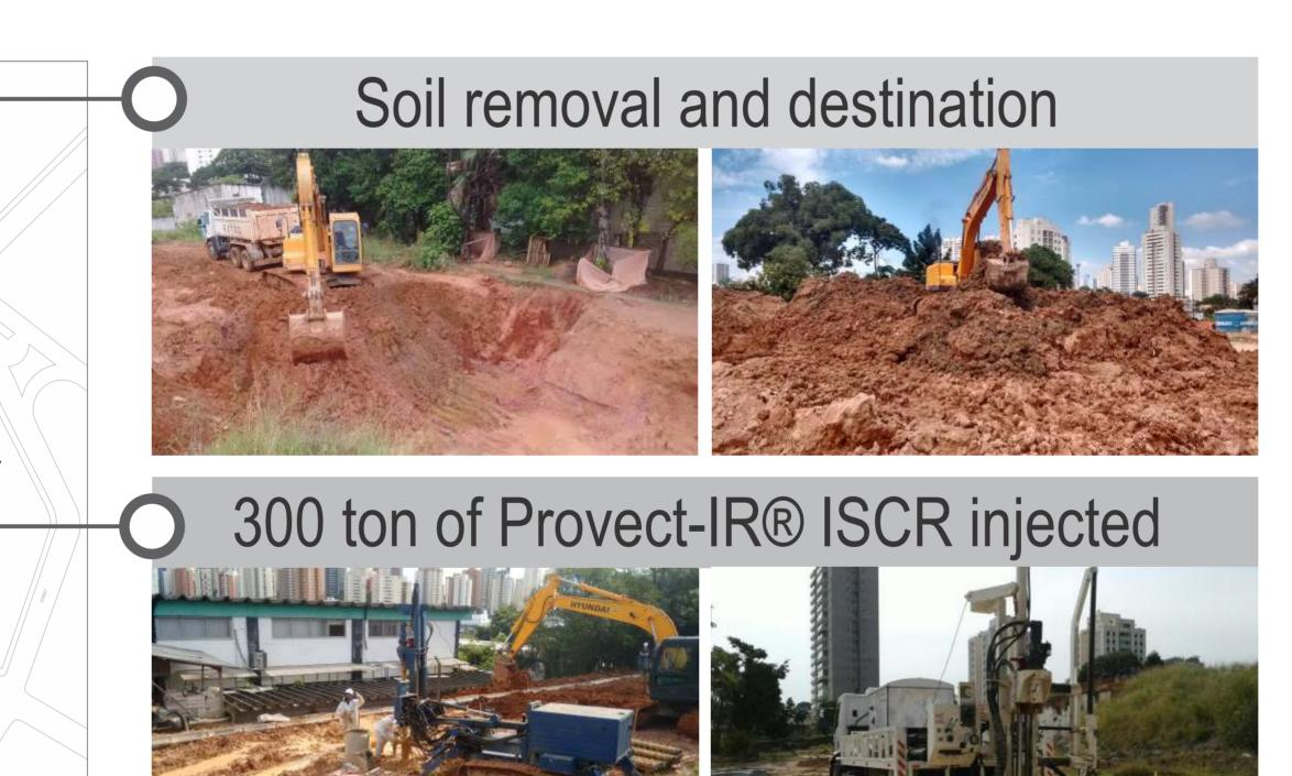
The field scale remediation included the removal and off-site disposal of 24,300 ton of contaminated soil (mainly clay, in which ISCR wouldn't be effective) and in situ groundwater treatment through the injection of 300 ton of antimethanogenic Provect-IR® in 537 points with multiple injection layers, due to contaminant distribution. Monthly measurements of pH and ORP were performed to evaluate the formation of the reactive zones.
